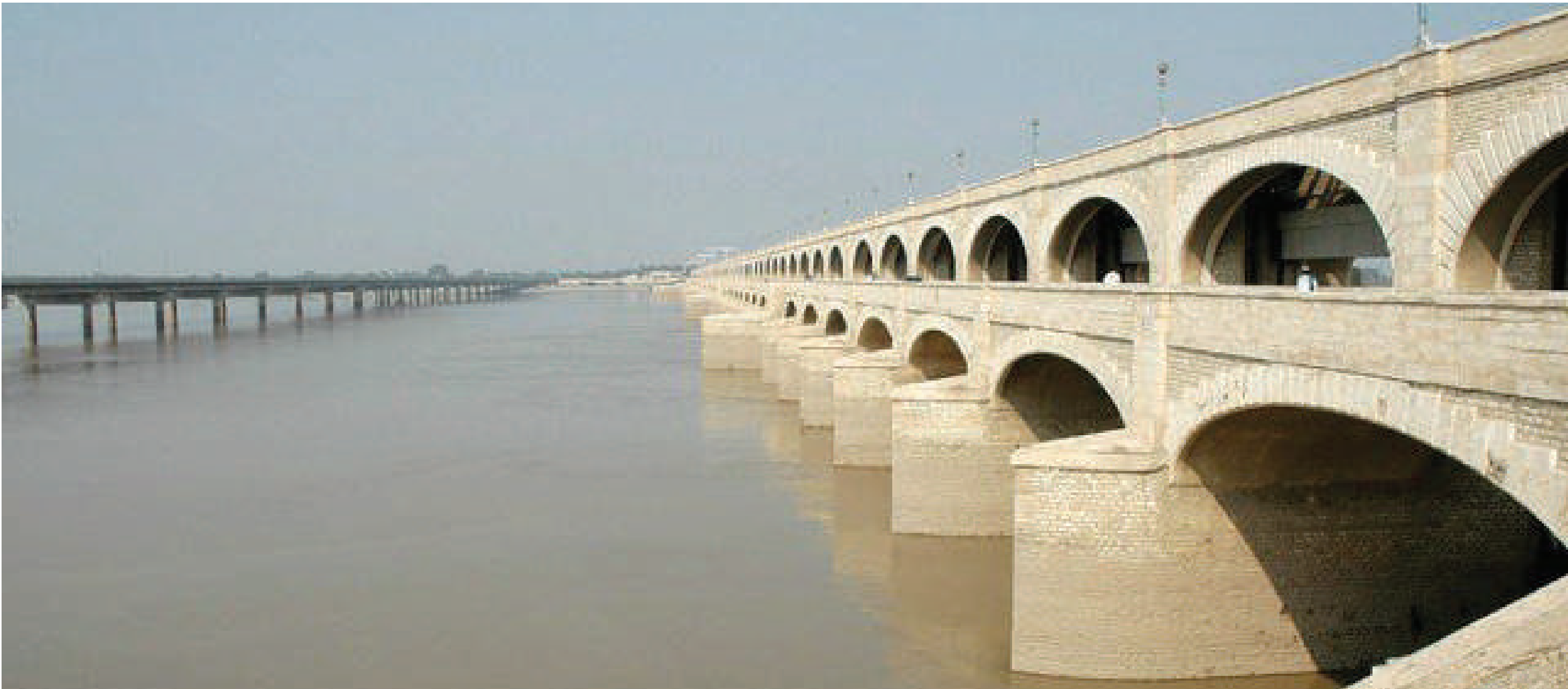
Image Source: http://tribune.com.pk/story/576922/provincial-initiatives-cm-plans-rehabilitation-of-sukkur-barrage/
